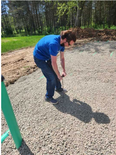
Photo depicts Public Health Sanitarian, Michael Grey, checking sand for depth compliance in a septic system's absorption bed.
